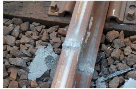
Track rehabilitation (including joint welds such as this one) result in a smoother, safer ride for customers.
