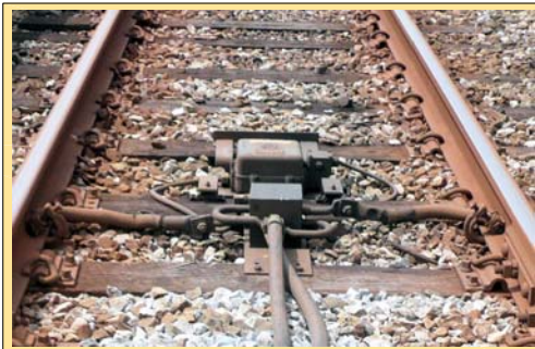
TYPICAL IMPEDENCE BOND (W Z BOND, OR "WEE-Z" BOND)
