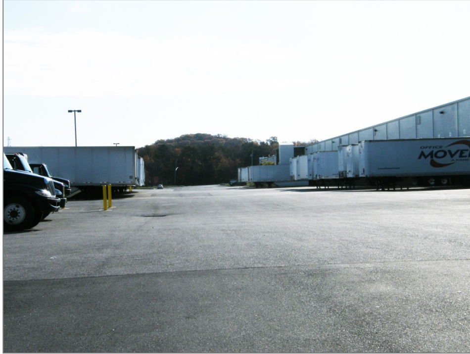
Figure 8. Partial view of warehouse adjacent to 3636 Pennsy Drive to the north (on the right)
