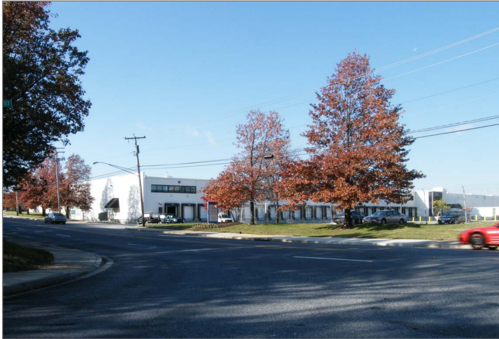
Figure 4. 3636 Pennsy Drive, south and east facades.
