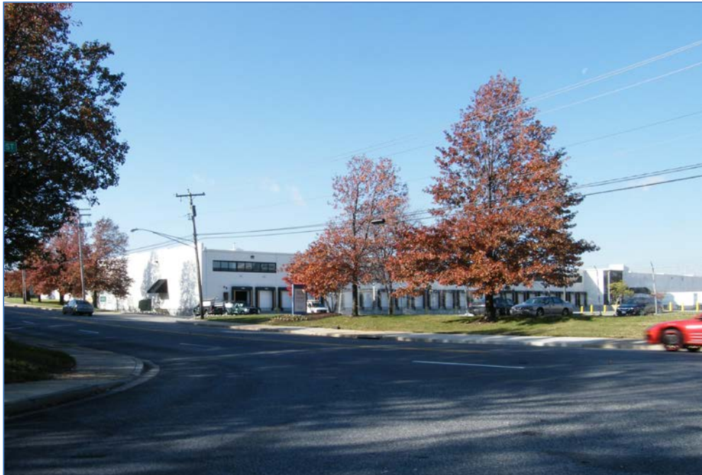
Photograph 1. 3636 Pennsy Drive, south and east facades. Nov. 12, 2014
