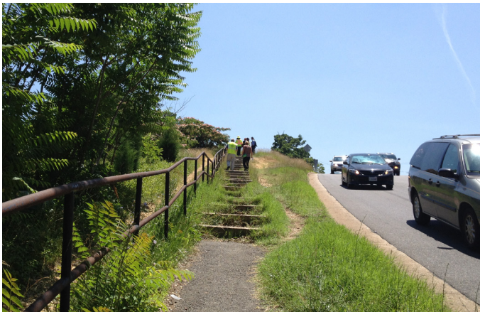
Figure 13 No ADA Provisions along South Van Dorn Street
