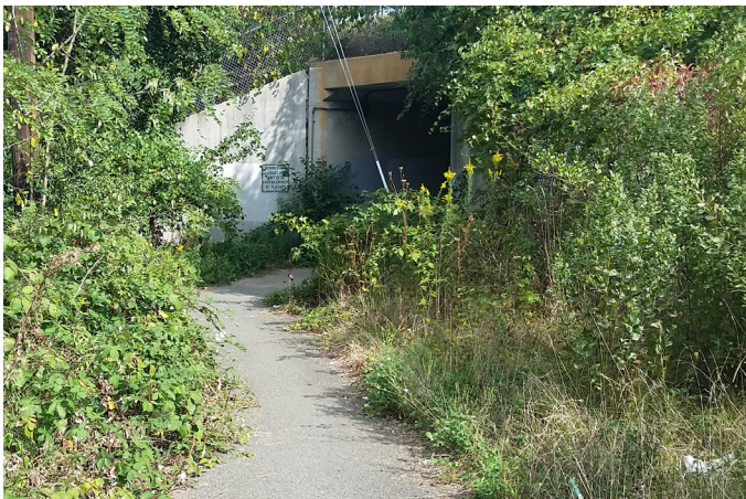
Figure 15 Overgrown Vegetation along South Van Dorn Trail
