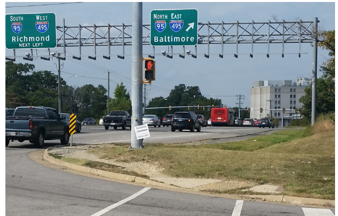
Figure 14 Inadequate ADA Provisions at Oakwood Road
