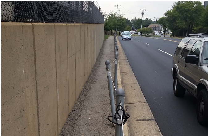
Figure 10 Narrow Sidewalk on Eisenhower Avenue near Metro Road
