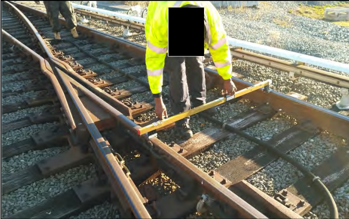
Checking gauge and cant at frog heel
