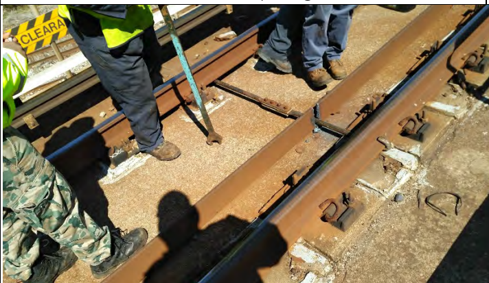
Completed Gauge Rod Installation
