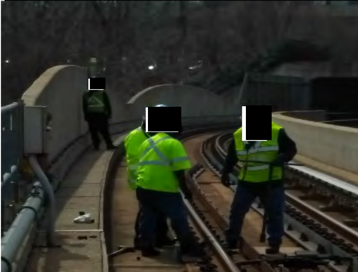
Maintenance Crew Completing Repairs
