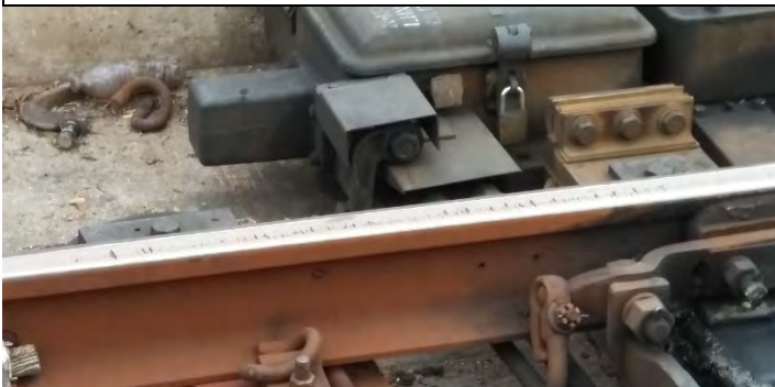
Rail Head Fatigue
