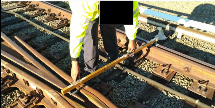
Checking flangeway gap at frog point (Diverging side)
