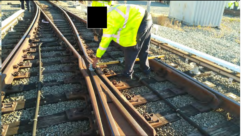
Checking flangeway gap at frog point (Straight side)
