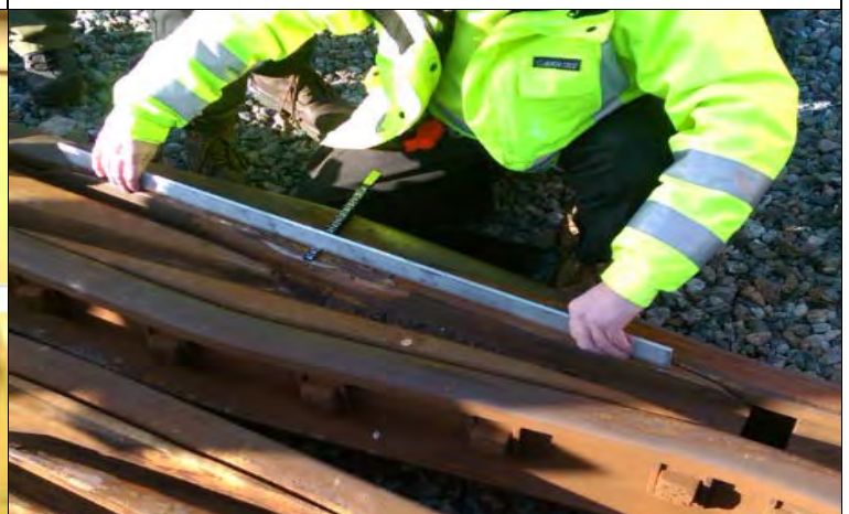
Figure 6: Riser Wear Measurement (Date: 03/29/17 Time: 0844)
