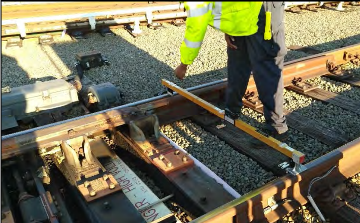
Checking gauge and cant before points
