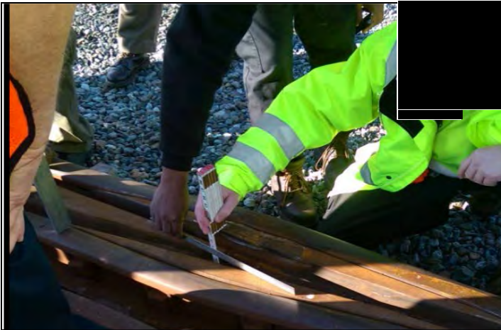
Figure 7: Flange-way Depth (Date: 03/29/17 Time: 0851)
