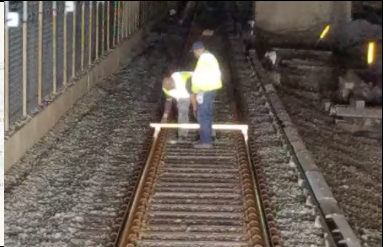
Measuring Narrow Gauge (03/09/17) – Photo 2
