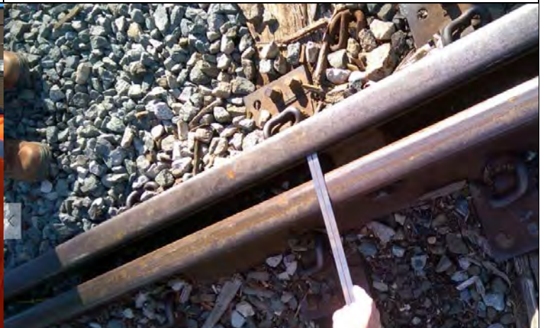
Figure 10: Guard Rail Opening Measurement (Date: 03/29/17 Time: 0934)
