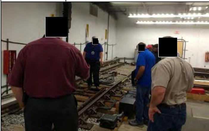
Full-Scale Demonstration on Turnout Inspection (B122)
