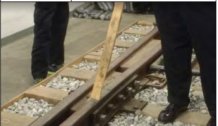
Explaining the Importance of the First Bolt on the Heelblock
