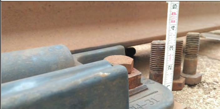
Short anchor bolts (Min 3.5" bottom of head to end)
