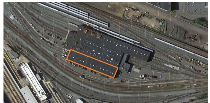
Aerial view. MRO highlighted (Washington, DC).
