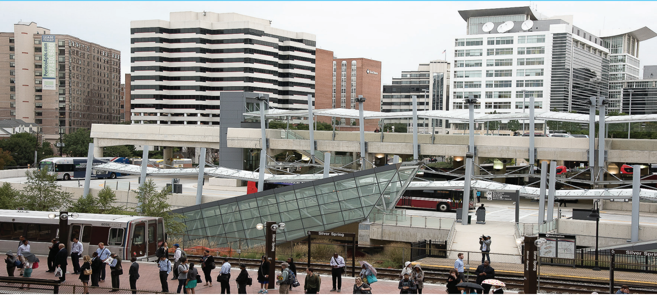
Compact urban development at the downtown Silver Spring Metrorail Station and Paul S. Sarbanes Transit Center.
