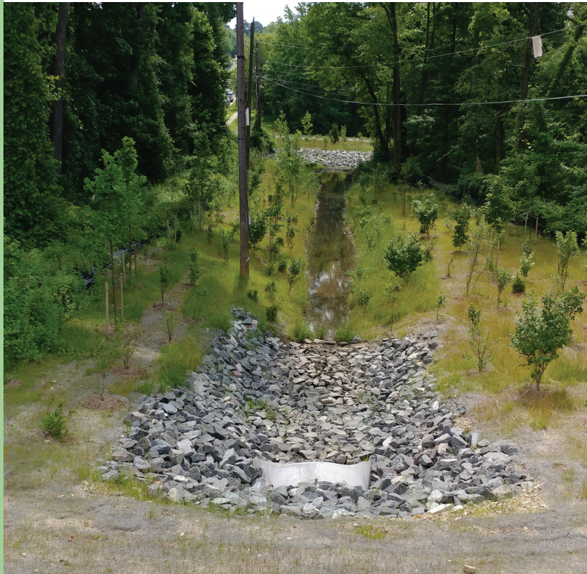
Stormwater treatment area at Cinder Bed Road Bus Garage can treat a 10-year storm at 66 cubic feet per second of stormwater.
