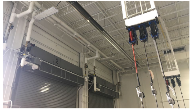
Andrews Federal Bus Garage reduces energy use through energy efficient features such as infrared gas heating and blower curtains.
