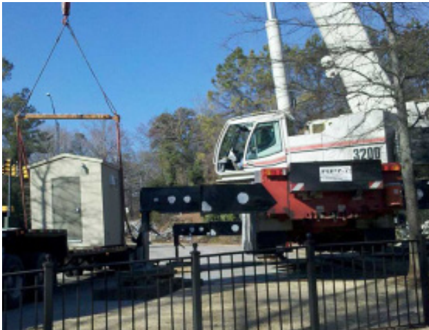
Prefabricated restroom crane installation
