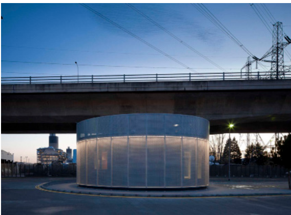
Daggenham Bus Facility Hub, East London, UK
