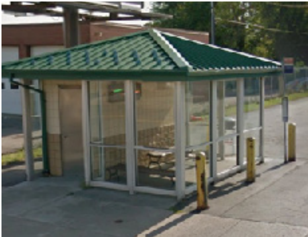
Buffalo, NY bus shelter and restroom
