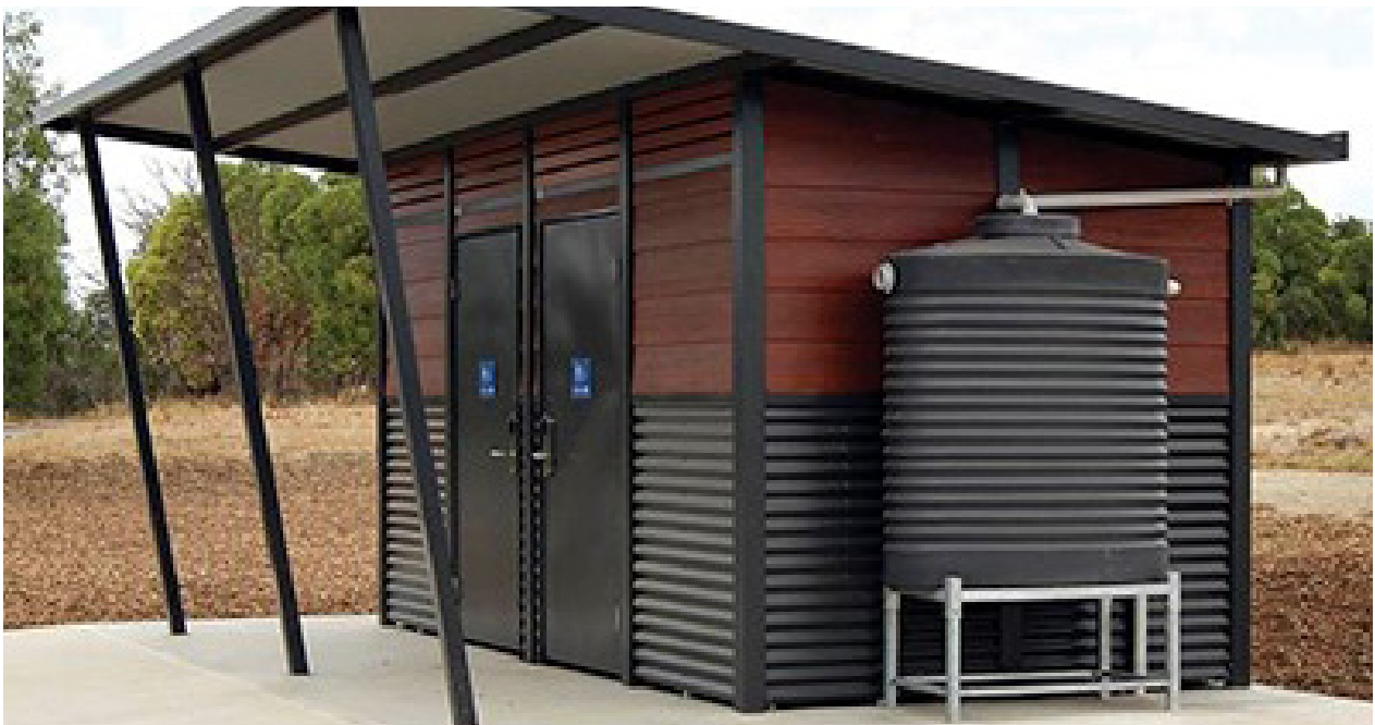
Waterless double restroom with rainwater tank, in Australia
