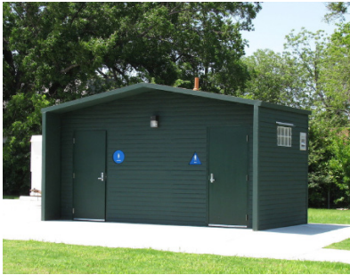
Modular connections restroom
