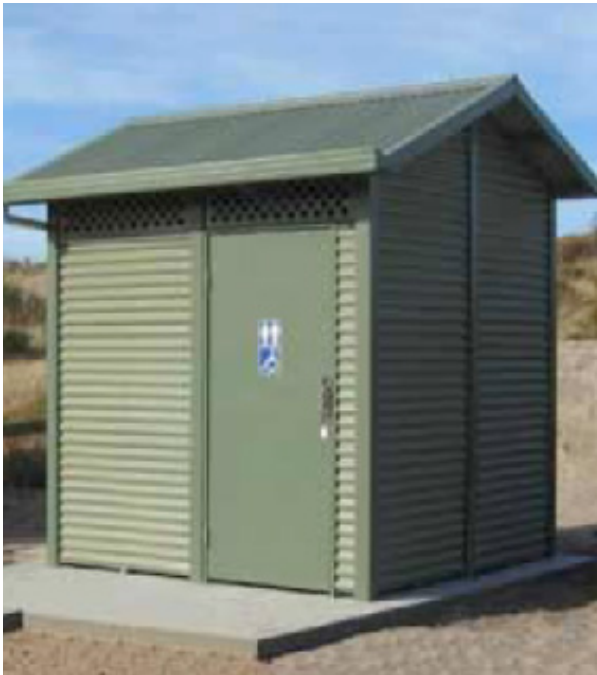
Prefabricated waterless single restroom
