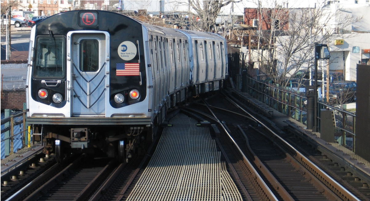
Figure 6 – NYCT Canarsie Line with CBTC Wayside Equipment on Right
