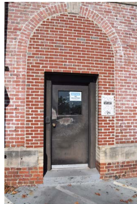
Window opening has been converted to a door
