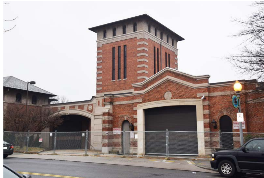
[Left] Administrative offices at north side; [Right] Tower with original entry at left and added entry at right
