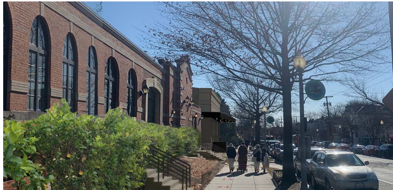
VIEW LOOKING SOUTHEAST ALONG 14TH STREET AT ENTRY
