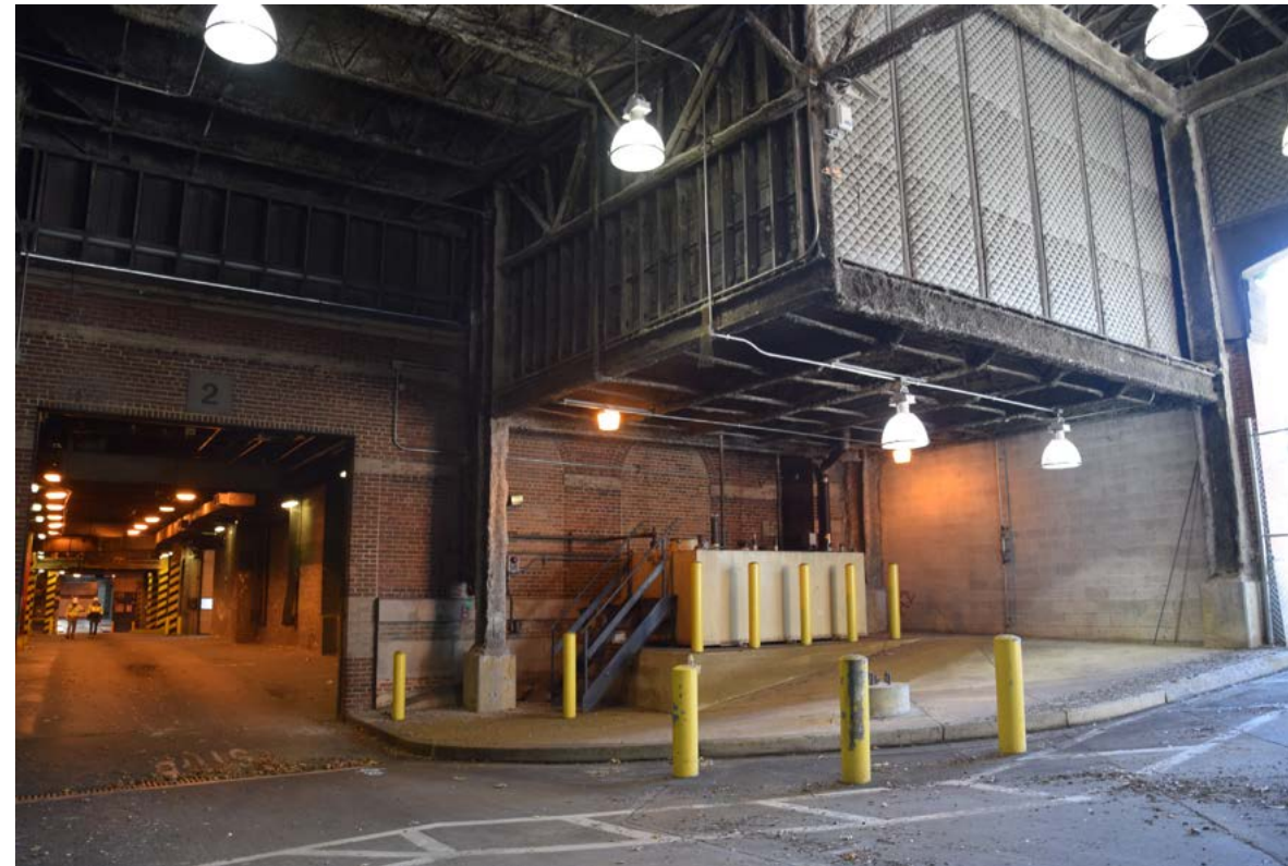
[Left] Original north elevation is currently enclosed and original windows have been infilled with brick; [Right] new bus openings have been added
