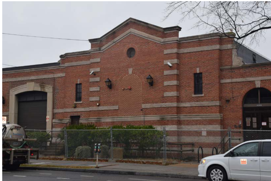
Southern end of west elevation; bus entry on left was added in 1987
