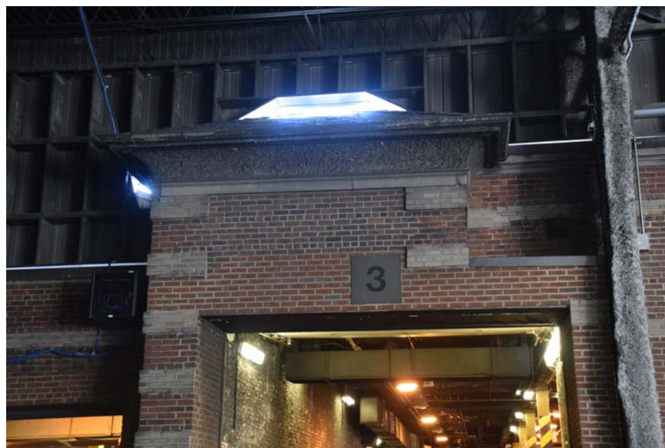
Hipped roof pavilion at north elevation
