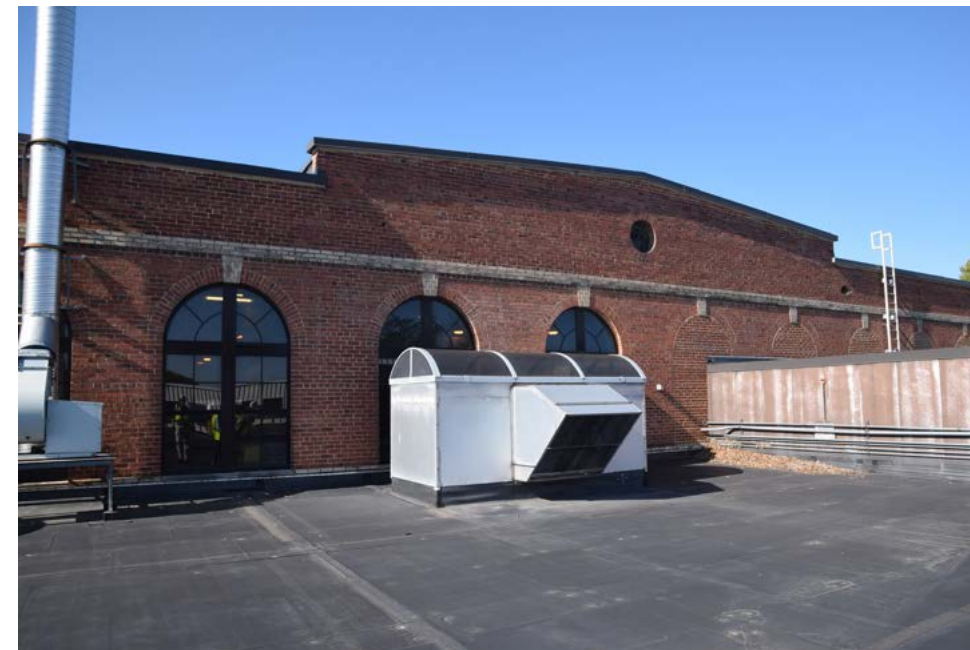
East Elevation Window openings have been infilled with brick
