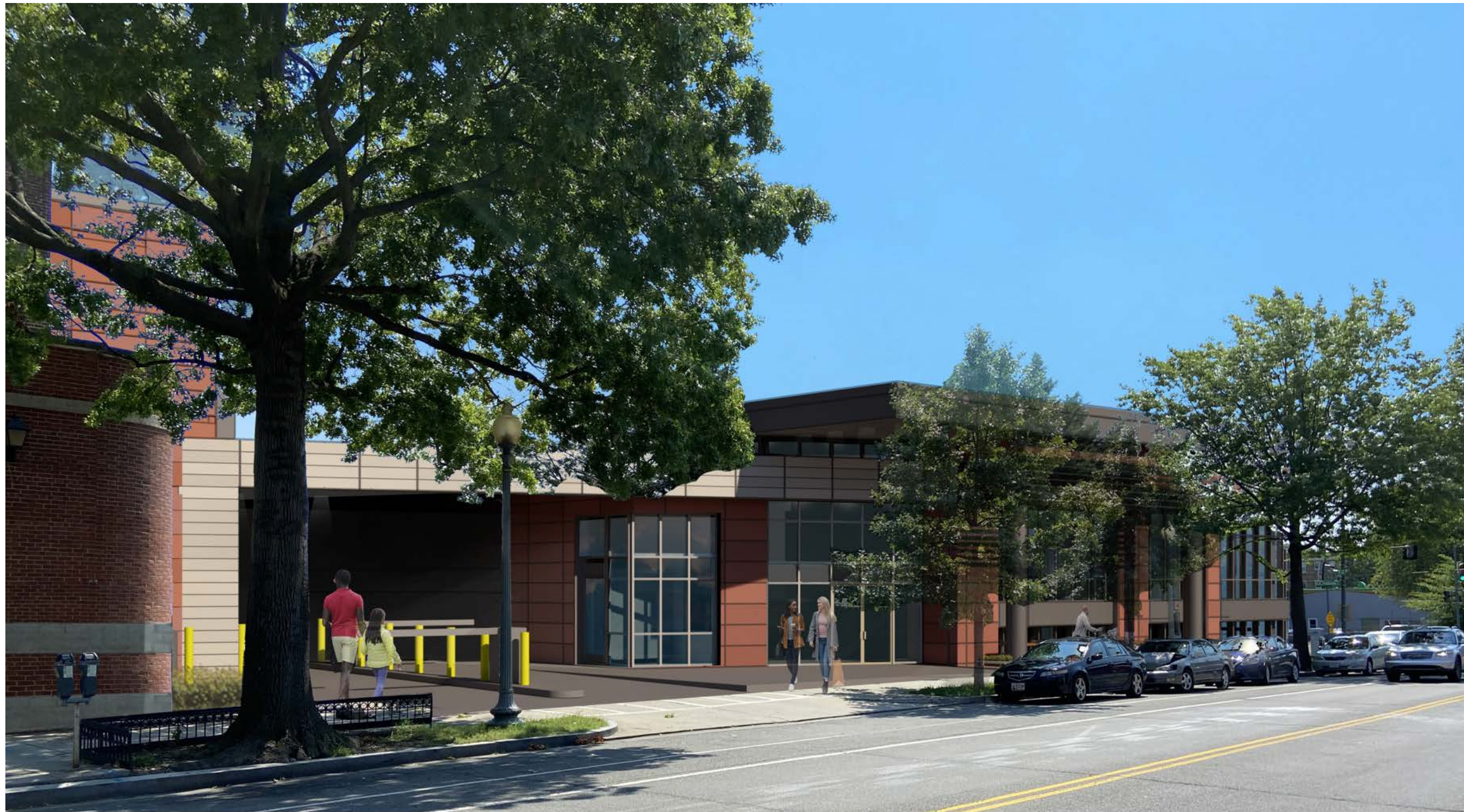
VIEW LOOKING SOUTHEAST ALONG 14TH STREET AT ENTRY
