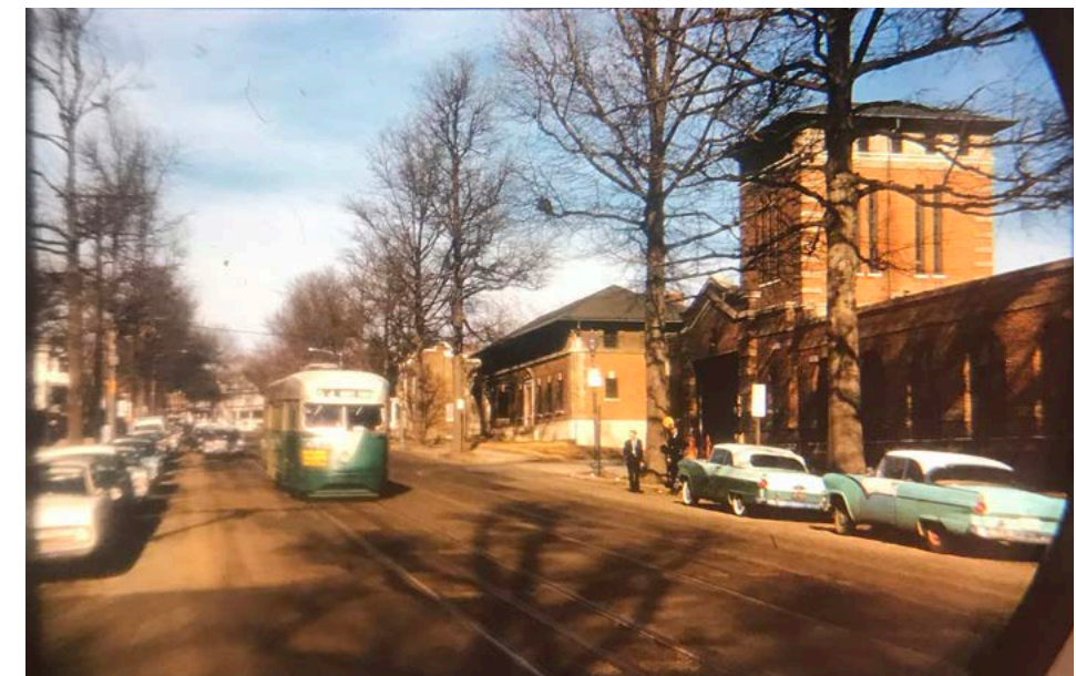
Car barn and tower, 1955-1962 (DC History Center)
