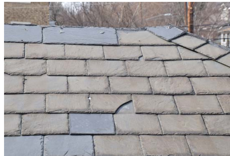
[Top] Cracked and spalling masonry surrounding an original street car barn opening; [Left] Slate roof of the administrative offices exhibits broken slates and inappropriate previous repairs; [Right] Stucco under the eaves of the administrative offices exhibits cracking and spalling
