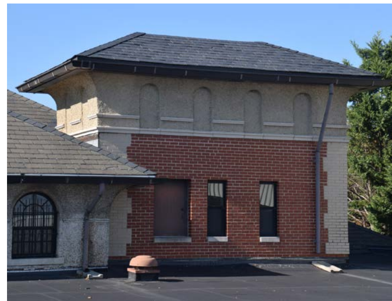
Non-historic stair and elevator tower, added 1987-1992
