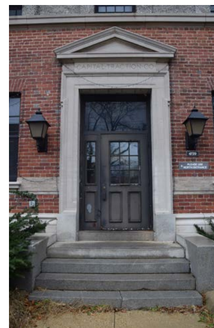
Door with original door surround at admin offices
