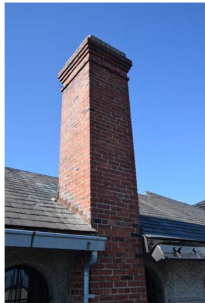
Admin offices chimney
