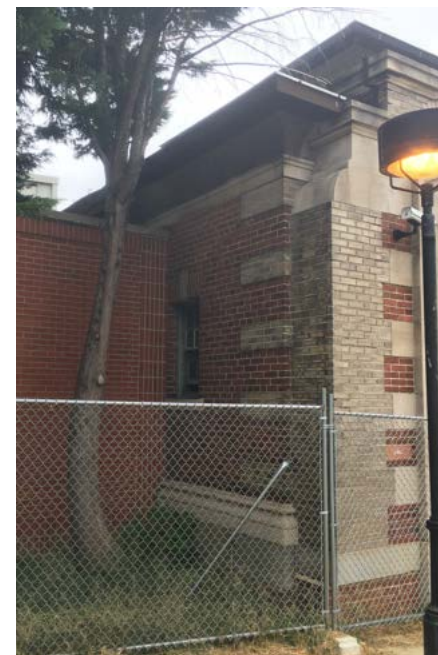
Original window extant on north side of admin offices
