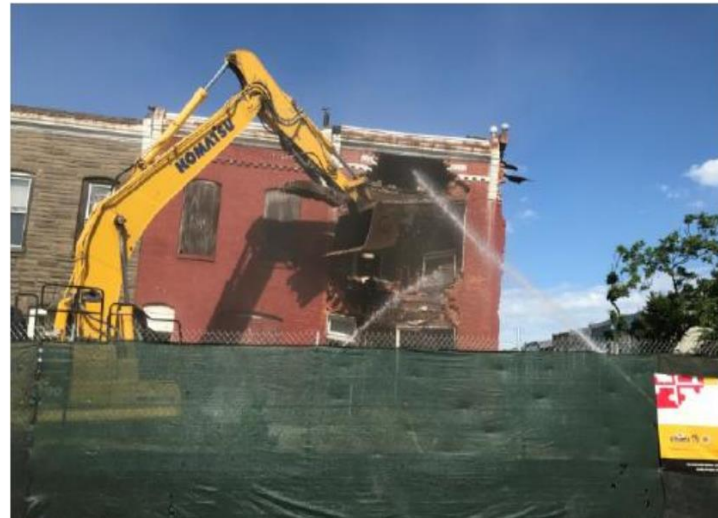
Maryland Stadium Authority – Project C.O.R.E.
