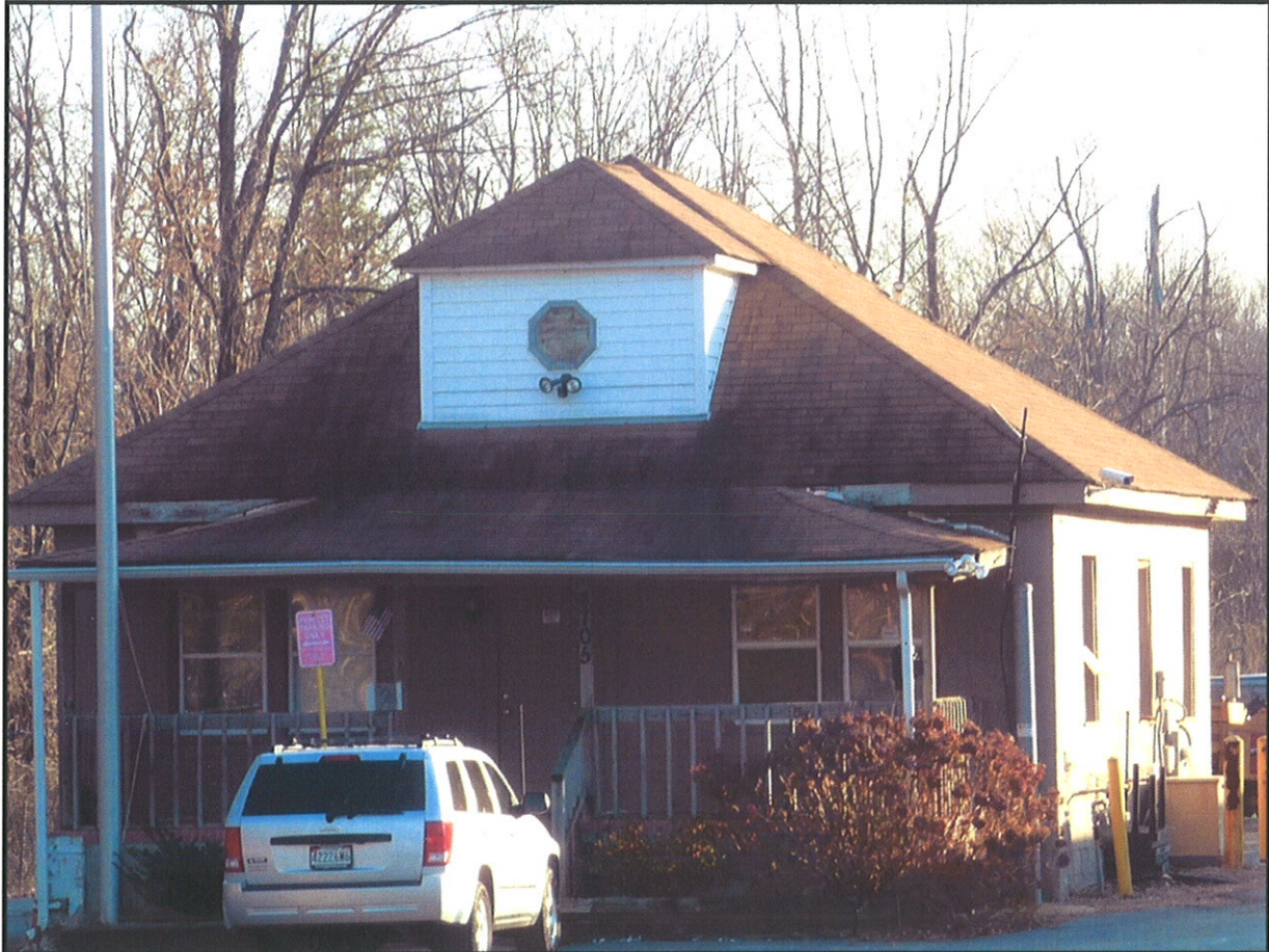
Photograph 1: View of 8705 Westphalia Road, looking south at main elevation. Note modern porch and balustrade, as well as heavily altered dormer. The residence has been converted into offices for the business in this location.
