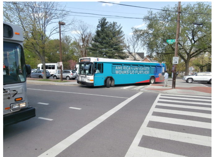
The uneven intersection of 40th Street, Fort Drive, and Albemarle Street NW causes awkward vehicular movements for cars and buses alike, putting pedestrians in harms way and increasing the likelihood of accidents.
