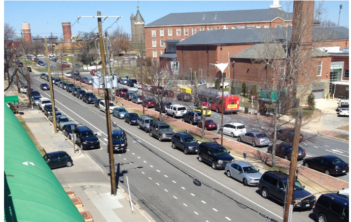
Overhead electrical wires and utility poles as seen along 40th Street in the project study area.
