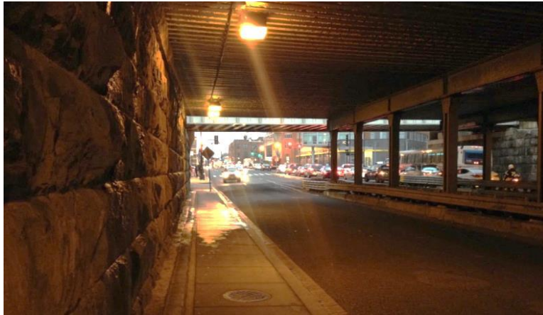
Figure 1: Narrow Sidewalk along Florida Avenue
