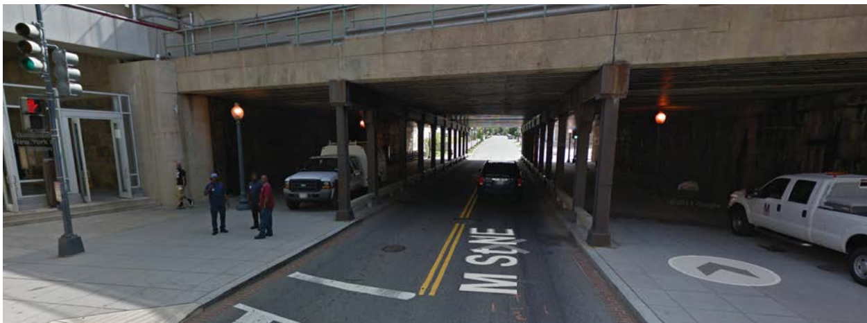
Figure 4: Wide Sidewalks in front of NoMa Metro Station South Entrance
