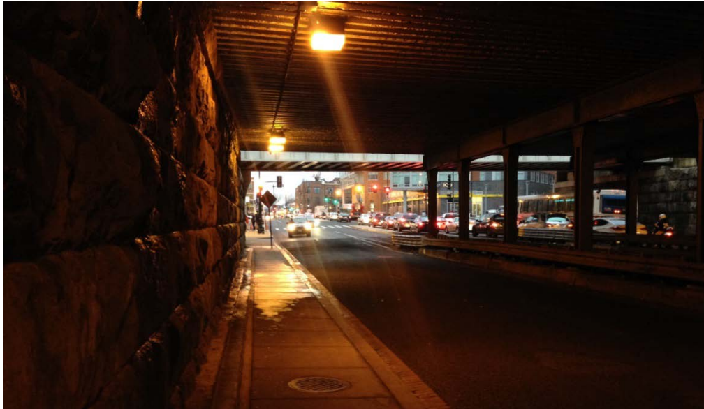
Figure 5: Narrow Sidewalk along Florida Avenue
