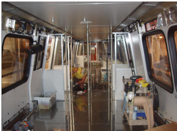
WMATA Railcar 3172 Being Rehabilitated in Hornell,
