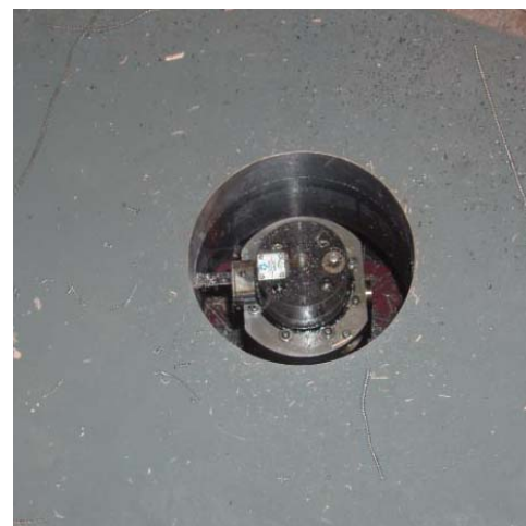
View of Top of Boring of Hole from Inside the Railcar
