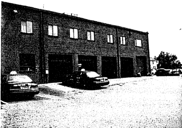
Arlington Maintenance Facility
