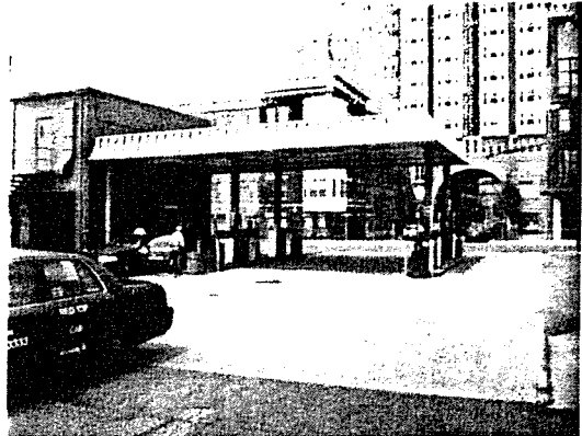
Arlington Fueling Facility
