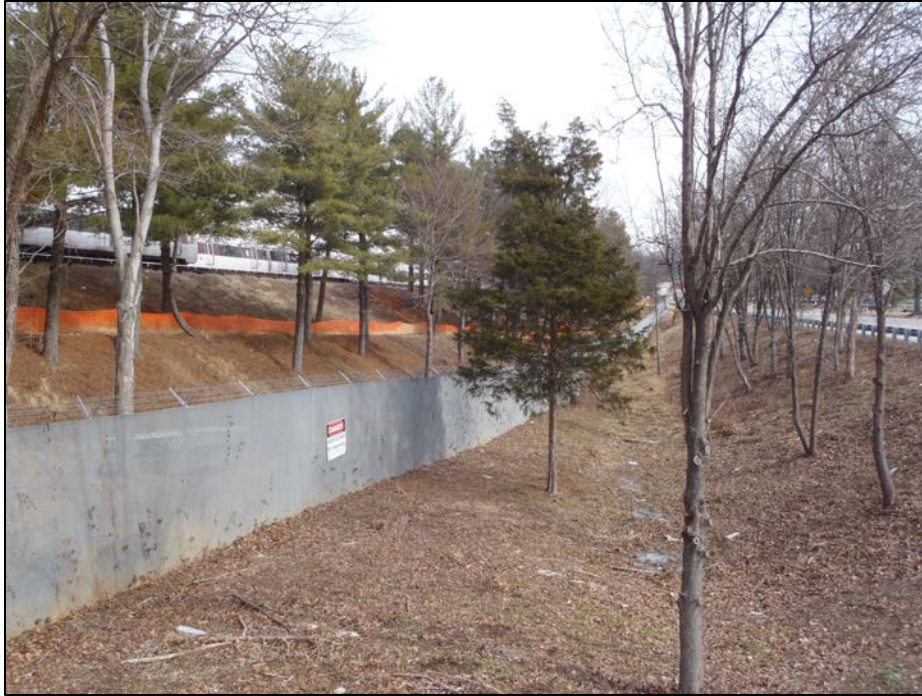
Photo 11. New Carrollton Yard, view northeast. This is the proposed location of the proposed contractor storage track and related access road and retaining wall. Garden City Drive is visible at the far right.
