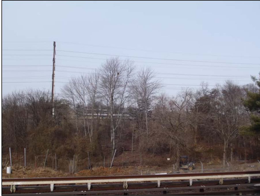
Photo 9. New Carrollton Yard, view northwest. The elevated Amtrak line is visible beyond the trees. New tracks of the north storage area would be level with the existing tracks in the immediate foreground.
