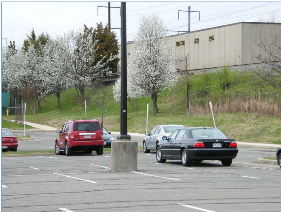
Photo 2. Landover Station, power traction facility, view west. Note high berm for rail corridor.
