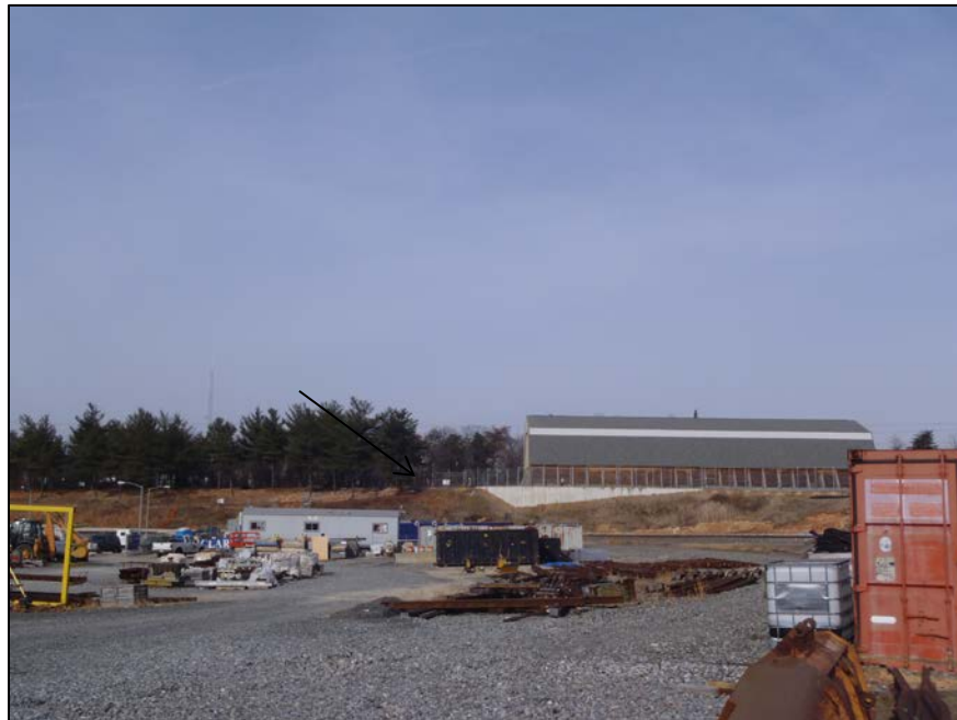
Photo 2. New Carrollton Yard, view northwest. The new parking lot, operations building for the northeast storage tracks, and stair/elevator/control tower would be located on this gravel area. The building on the embankment in the background is a SHA salt barn, outside the LOD but within the APE. The new operations building for the northwest storage tracks will be located to the left (southwest) of the saltbarn, on the embankment.
