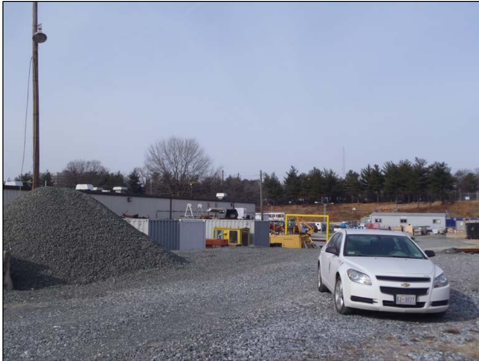
Photo 3. New Carrollton Yard, view southwest. The new northeast storage tracks and related operations building and parking lot would be located on this gravel area.
