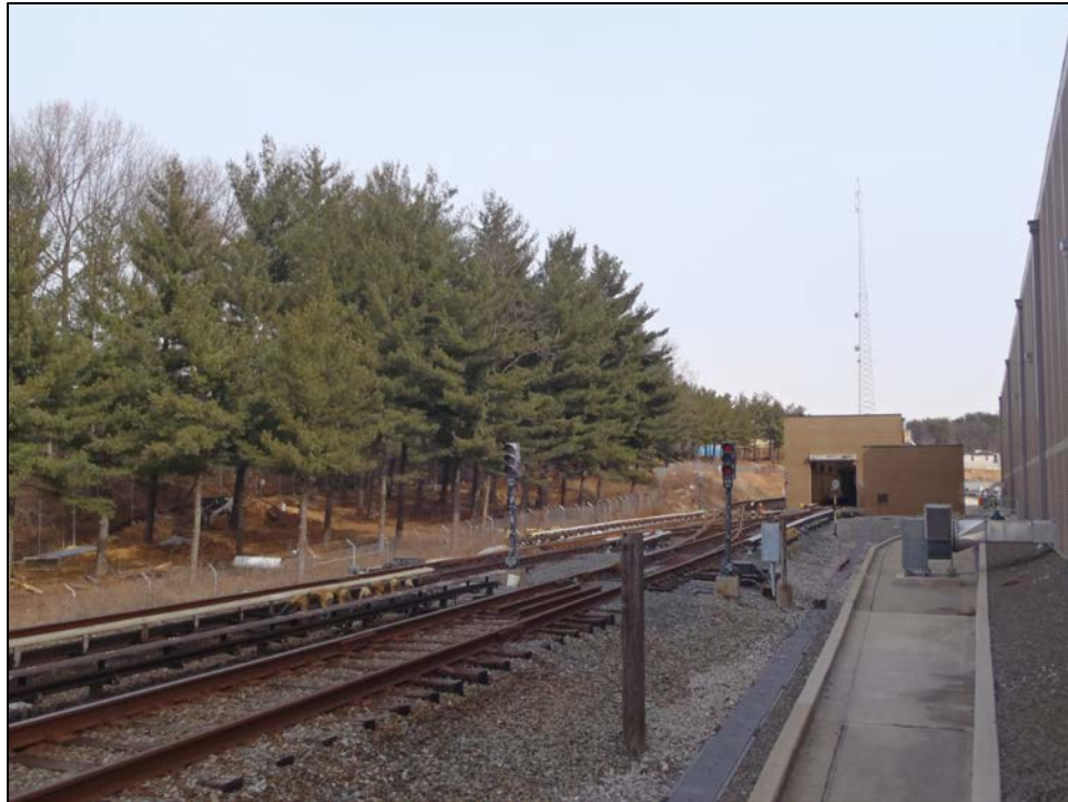
Photo 7. New Carrollton Yard, view northeast. The car wash building is visible at right. The wall of the repair shop, constructed circa 2004, is at the extreme right.
