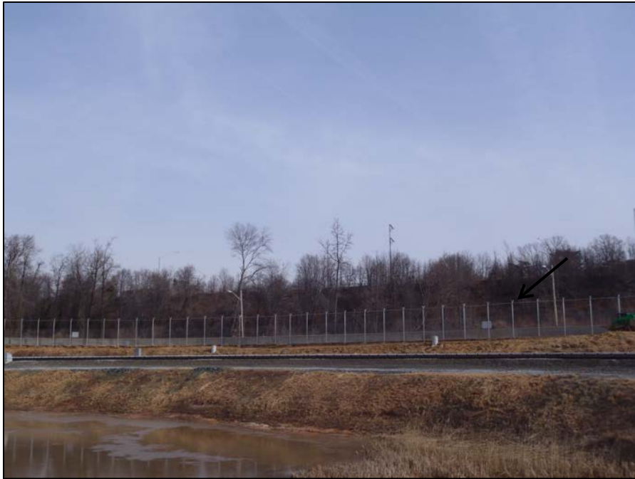
Photo 1. New Carrollton Yard, view north. The fence marks the edge of WMATA property, and the noisewalls for I-495/I-95 are visible beyond.
