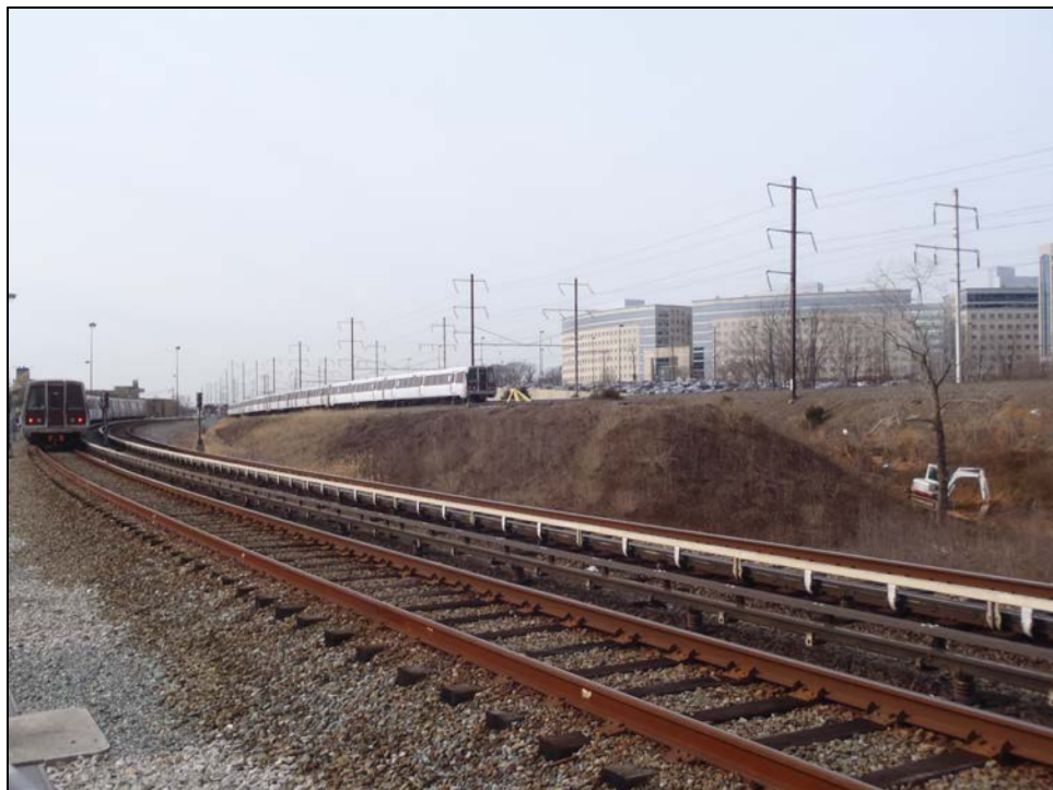
Photo 8. New Carrollton Yard, view southwest. The valley will be infilled and tracks will be laid to connect these tracks to the proposed northwest track storage area.
