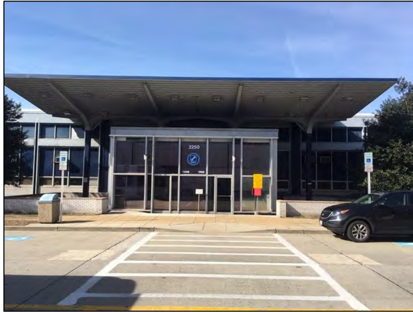
Figure 14: Building 1 North entrance Canopy and Portico, facing South
