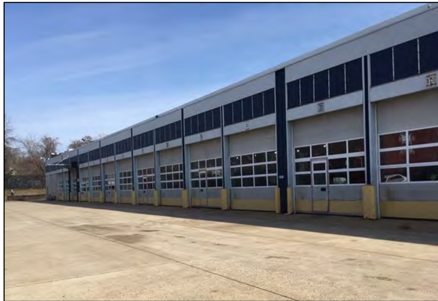
Figure 13: Building 1 South Elevation, facing Northwest
