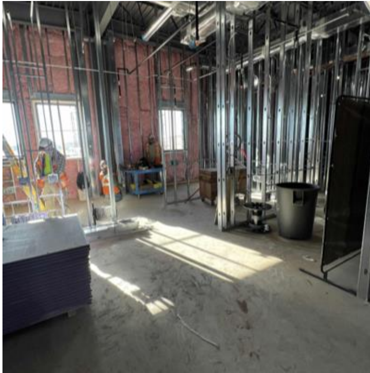
Level 2 Framing & Insulation
