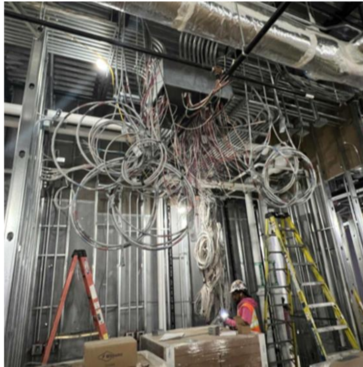
Electrical Wire Pulling
