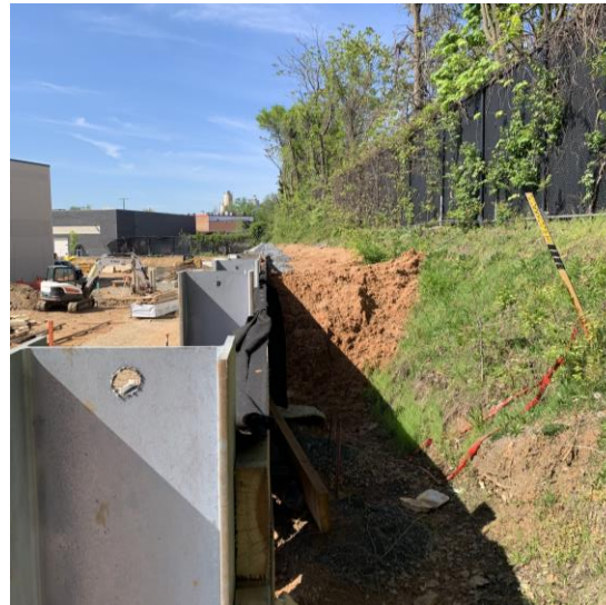
CSX Retaining Wall Install
