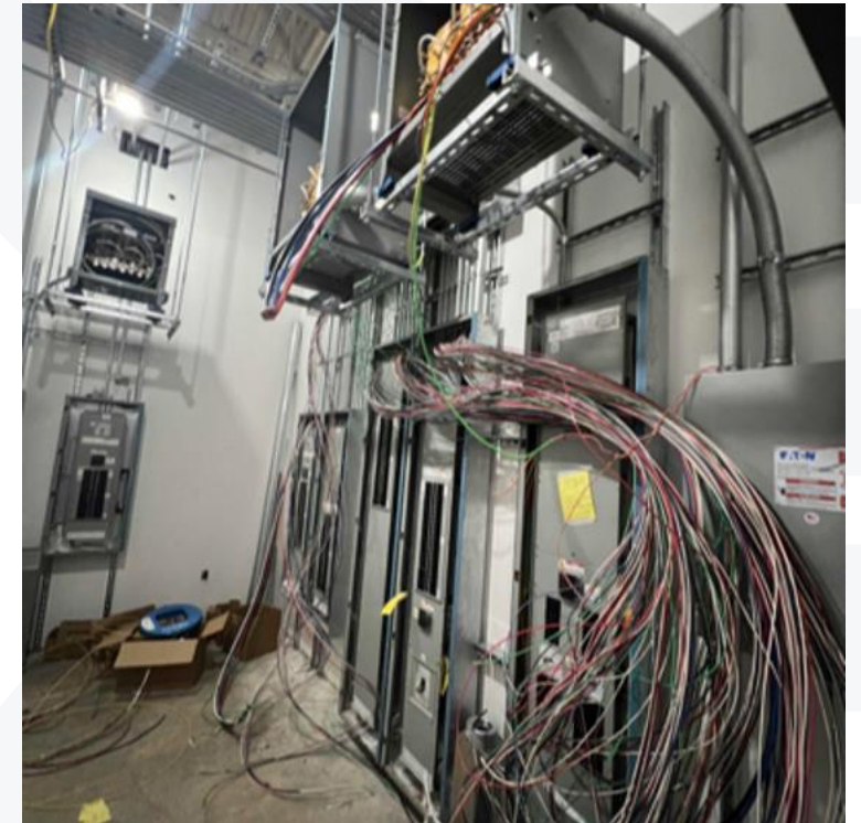
Electrical Room Wire Pulling
