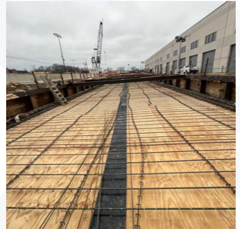
RWH 2-8 Lid Progress
