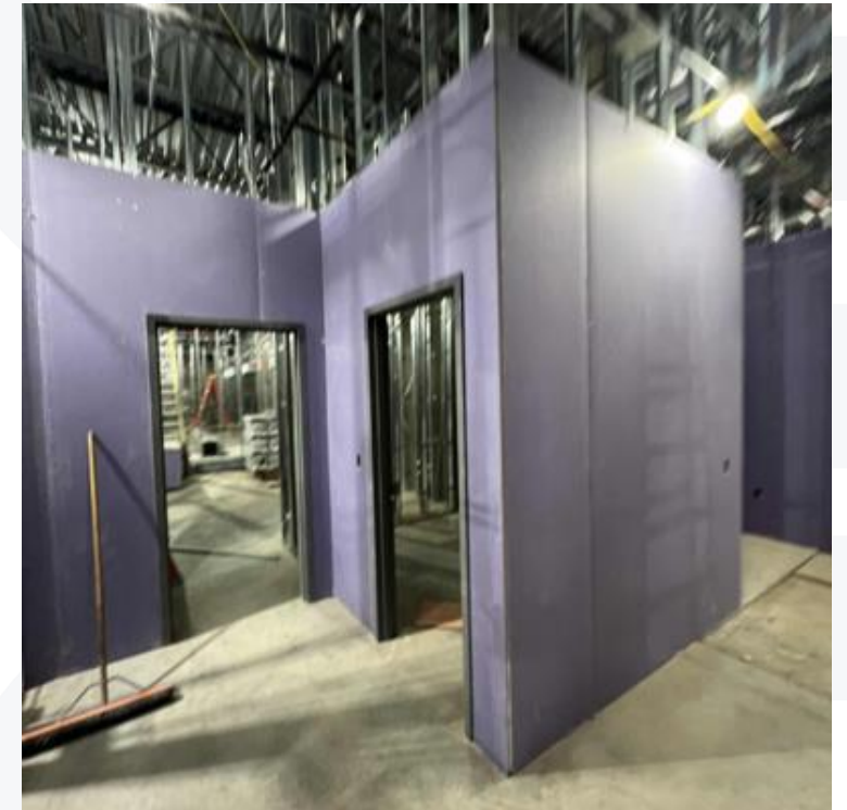
Level 2 Framing & Drywall
