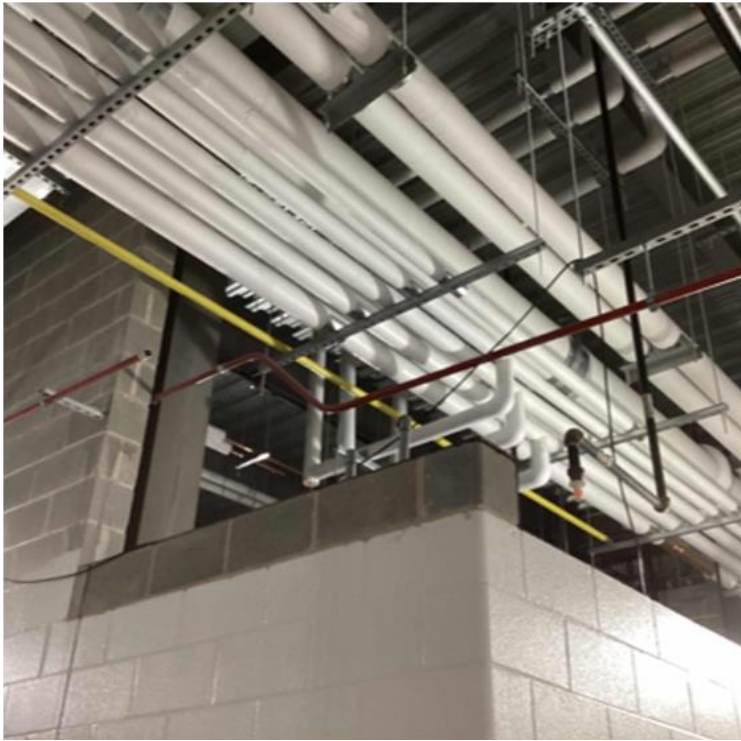
Mechanical Piping Tested & Insulated
