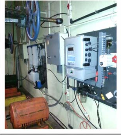
Seven chiller plants were fitted with state-of-the-art water treatment systems, saving an estimated 400,000 gallons of water per location annually.
