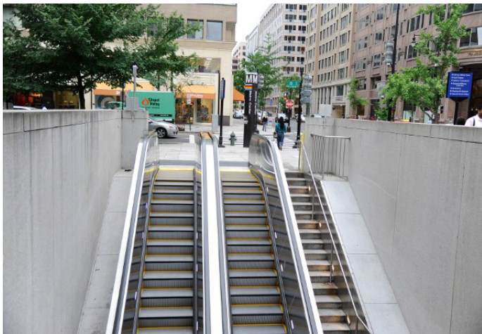
Metro is the single largest vertical transportation operator in North America.
