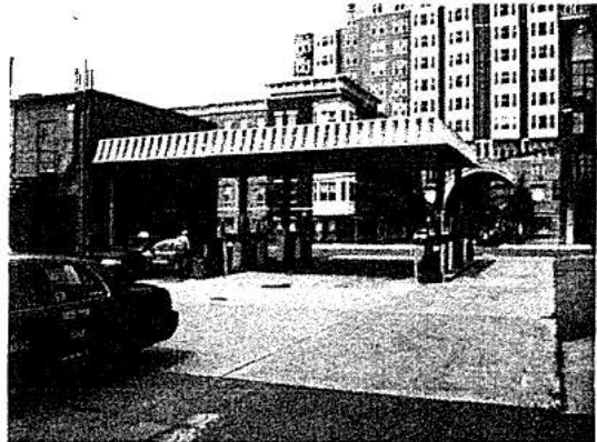
Arlington Fueling Facility
