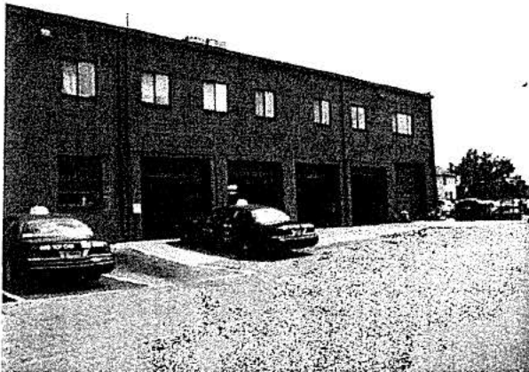
Arlington Maintenance Facility
